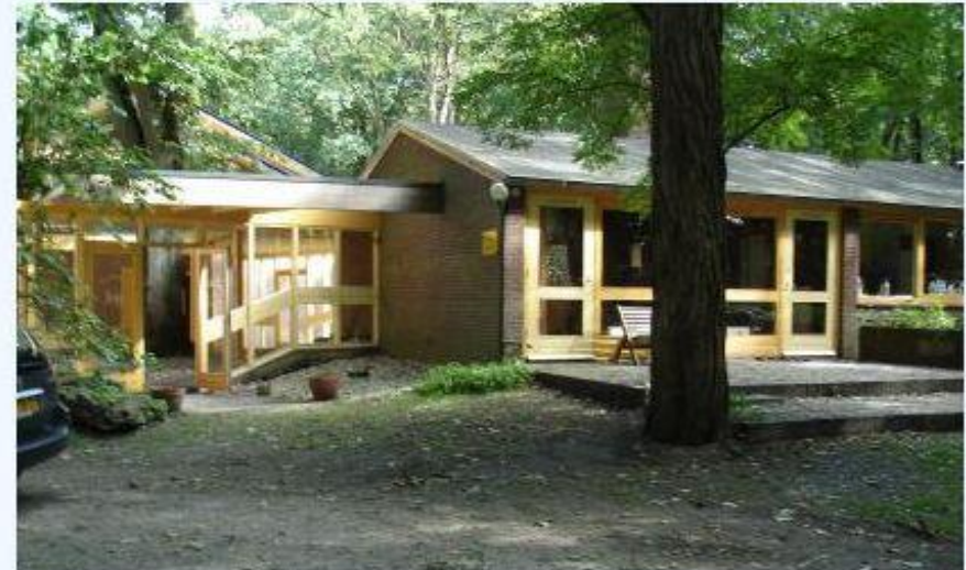
Arundale House on the right with entrance Crystal House and Hall on the left (2011)
