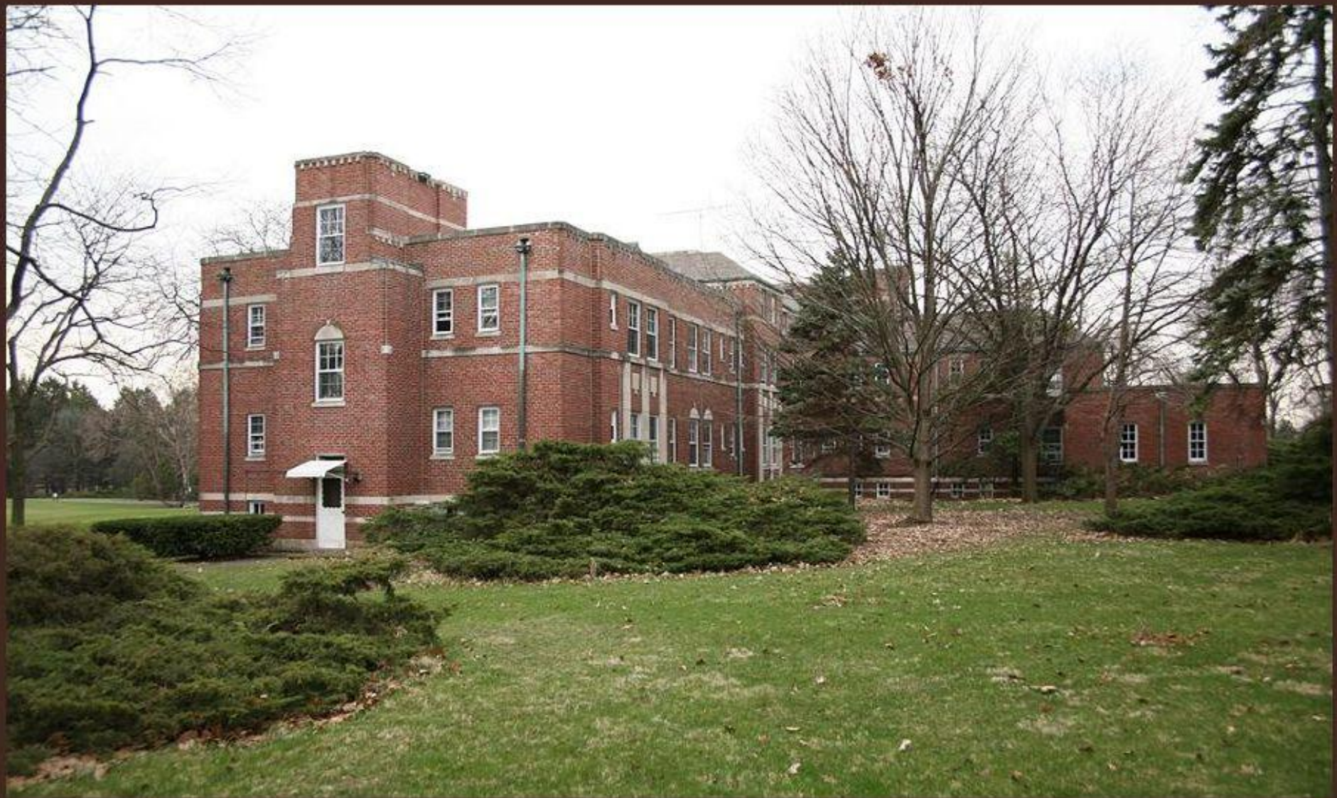
Building from North-West
