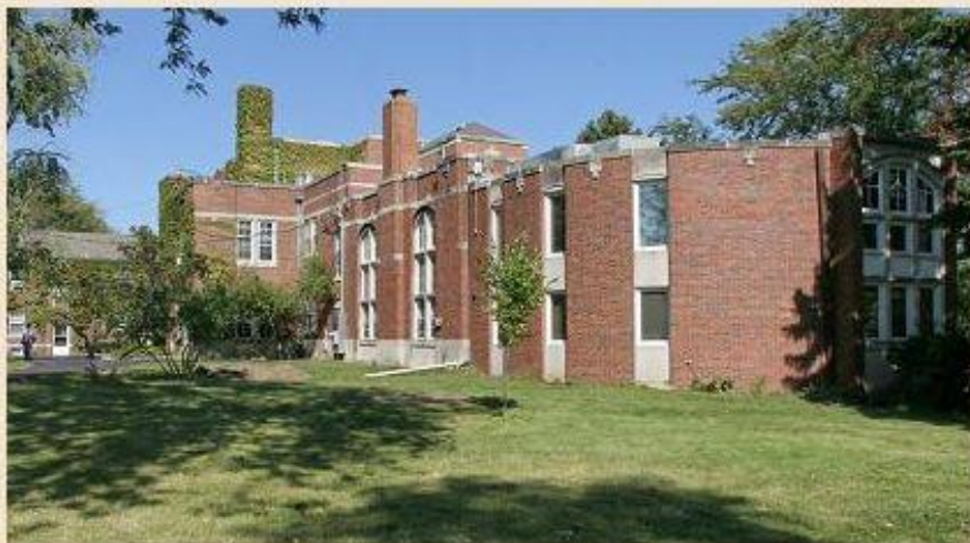
View of library wing from South-West
