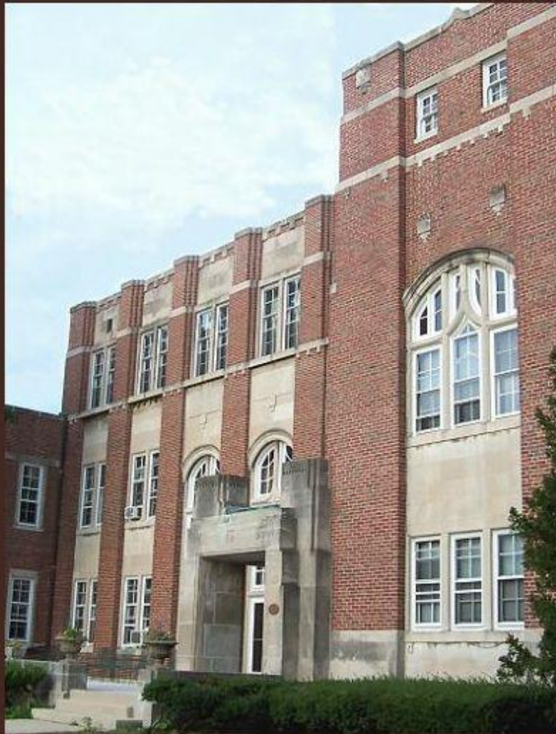
Front from North-East
