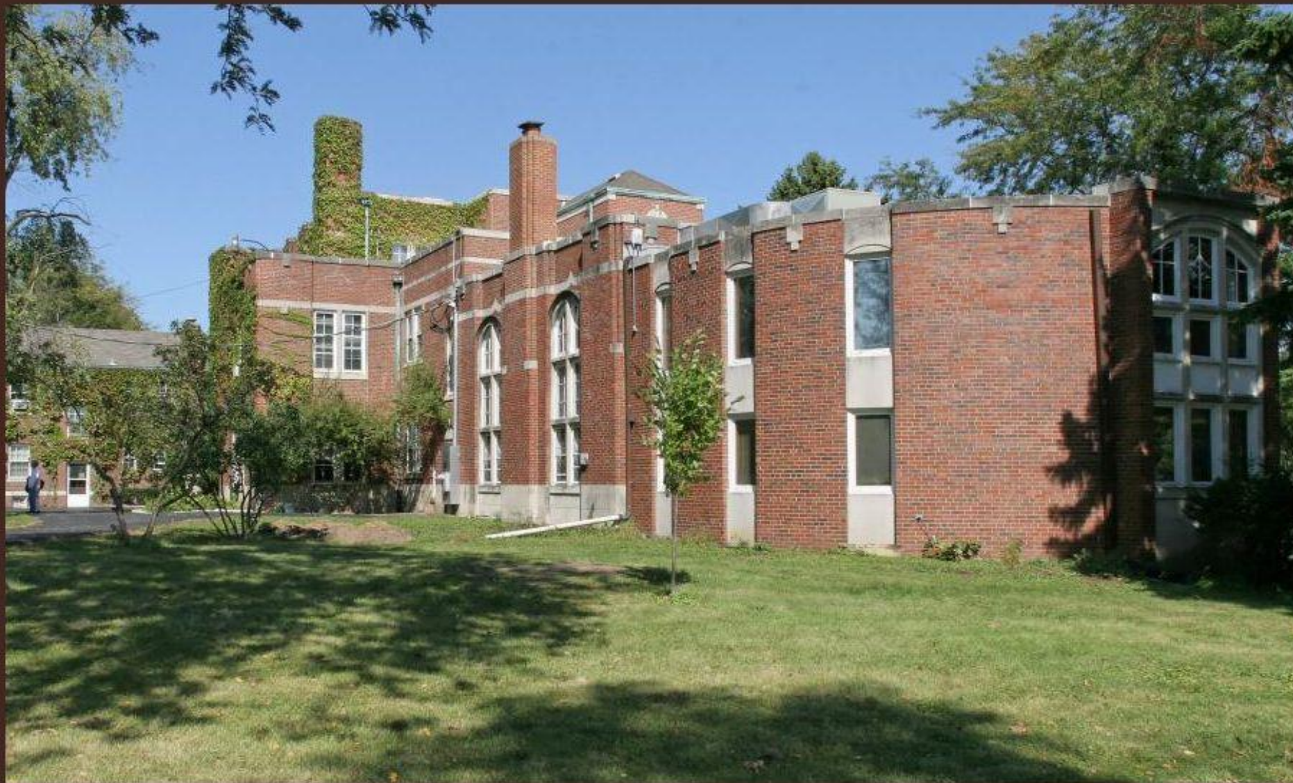
View of library wing from South-West
