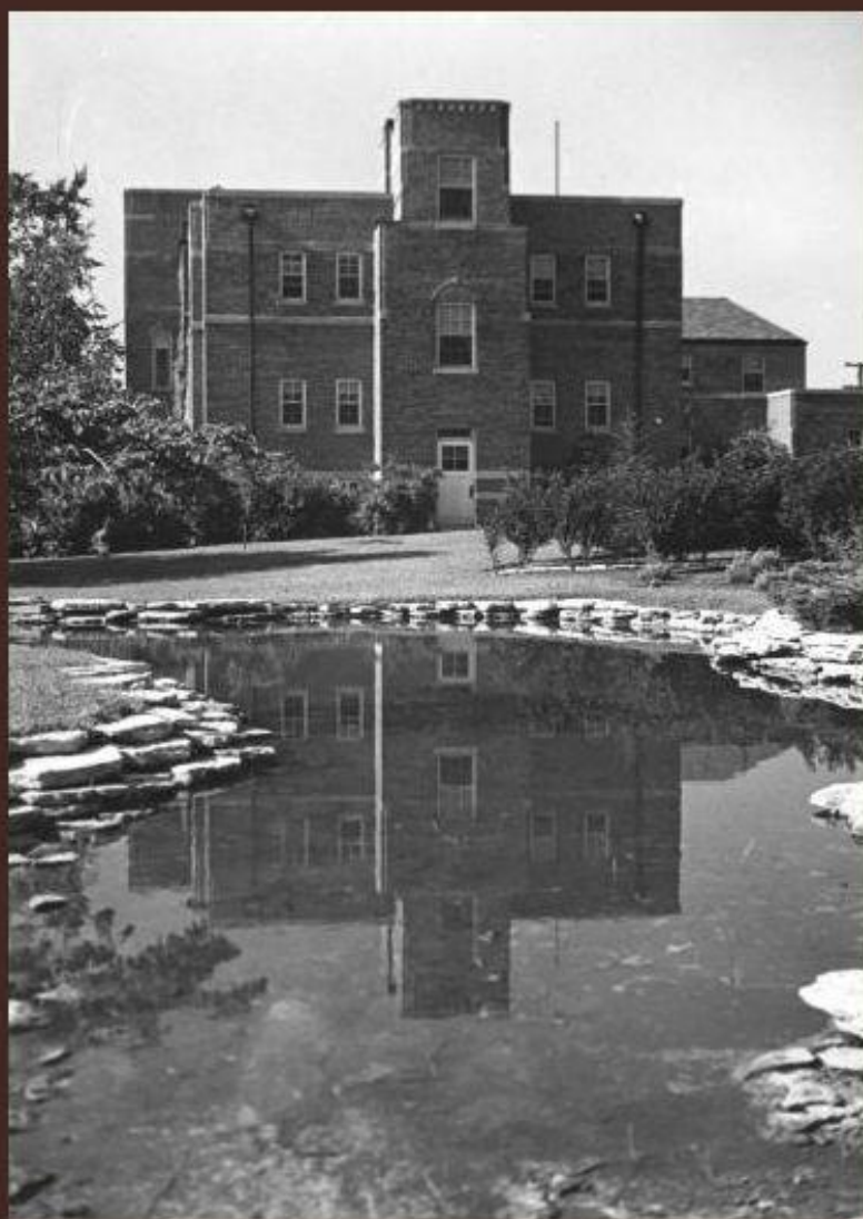
Building from North, 1938
