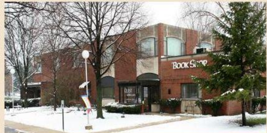
Mills Building exterior
