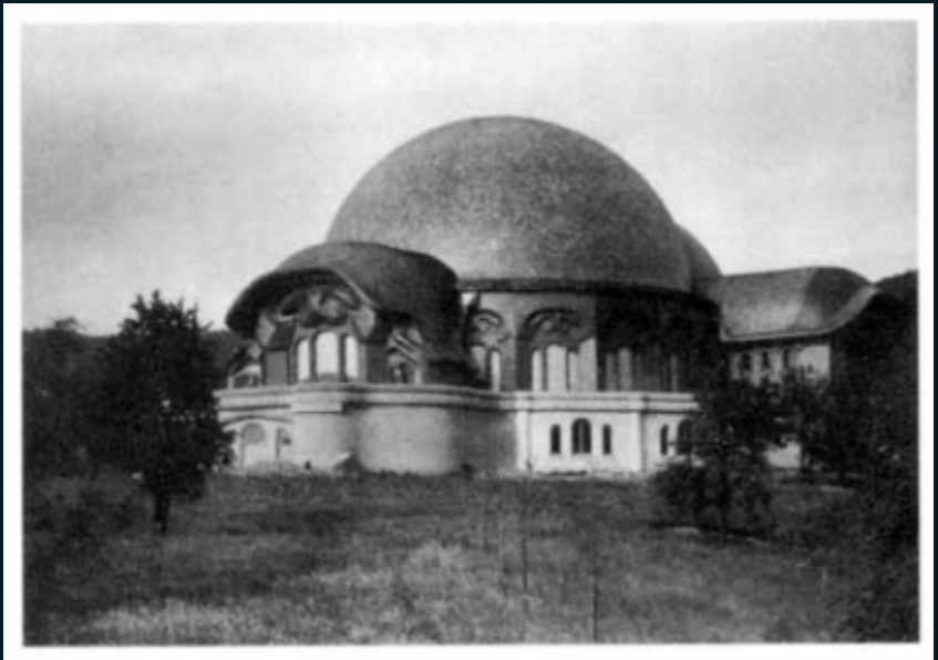
First Goetheanum - a timber and concrete structure designed by Rudolf Steiner
